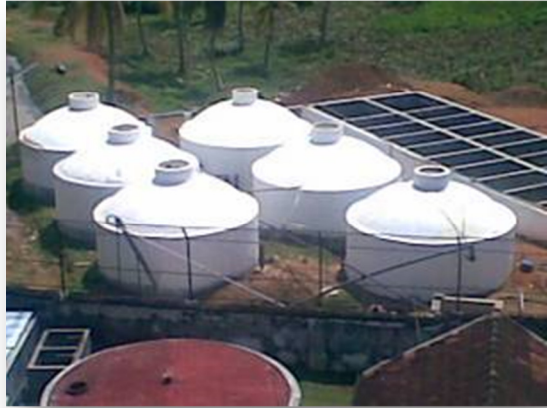
Wastewater treatment system (according to UAFF Biogas technology) of Sri Lanka Distilleries Ltd. - Wadduwa distillery , Wadduwa
