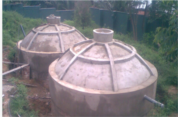
Wastewater treatment system (according to UAFF Biogas technology) of Rockland Distilleries Ltd. - Marawila Distillery , Marawila
