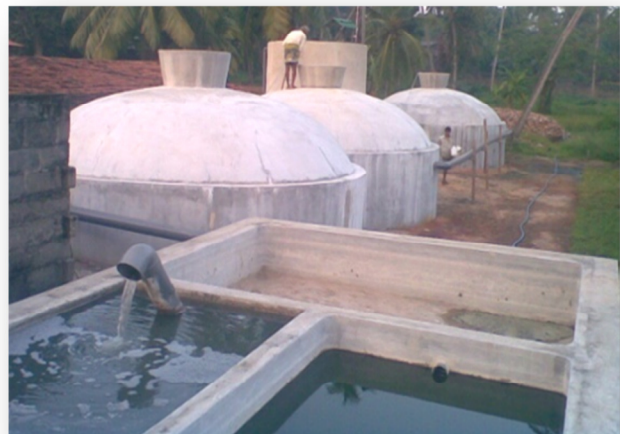
Wastewater treatment system (according to UAFF Biogas technology) of Minuwangoda D/C mills - Minuwangoda.
